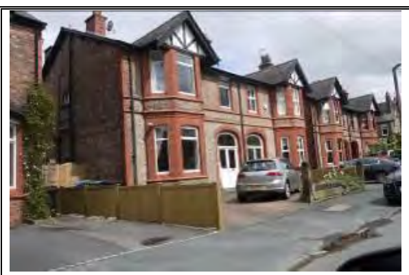
Photograph 26: Properties along Appleton Road
