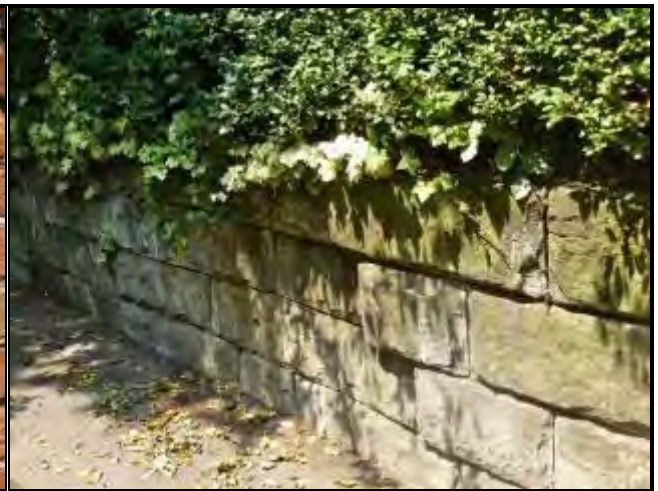
Photograph 122: Stone Wall on Harrop Road
