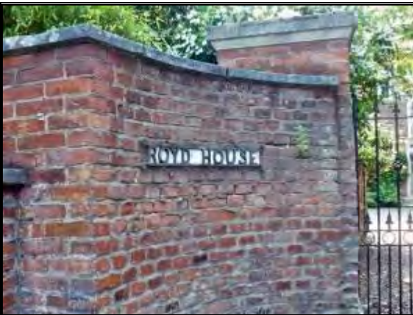
Photograph 80: Historic Brick Wall and Gate Pier, Park Road
