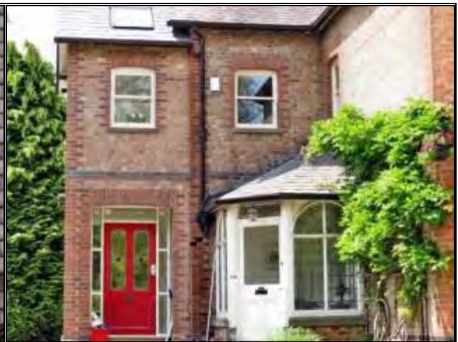
Photograph 110: New Entrance at 232 Ashley Road
