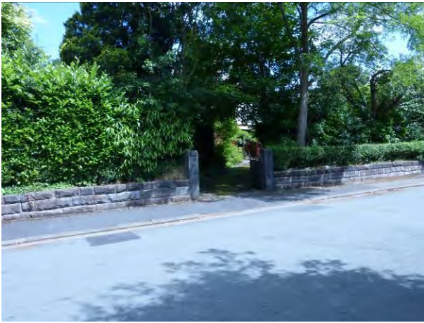
Original boundary treatment and gateposts
