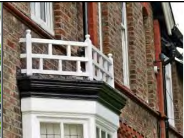
Photograph 19: Detail of Timber Railing on 2 Bower Road
