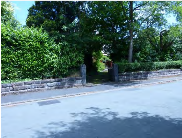
Original gateposts and low boundary walls
