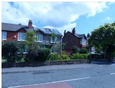
Solar panels on Arthog Road
