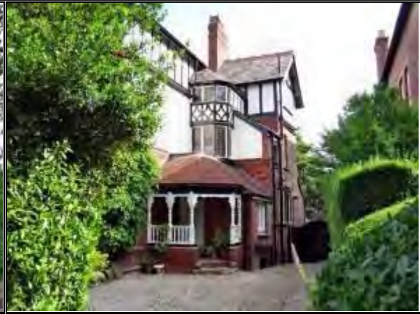
Photograph 17: Porch and Decorative Windows of 19 Park Road
