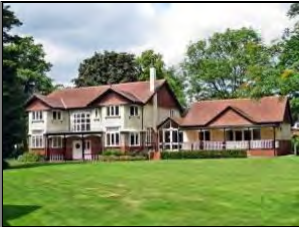
Photograph 36: Open Space between St. Peter's Church and House
