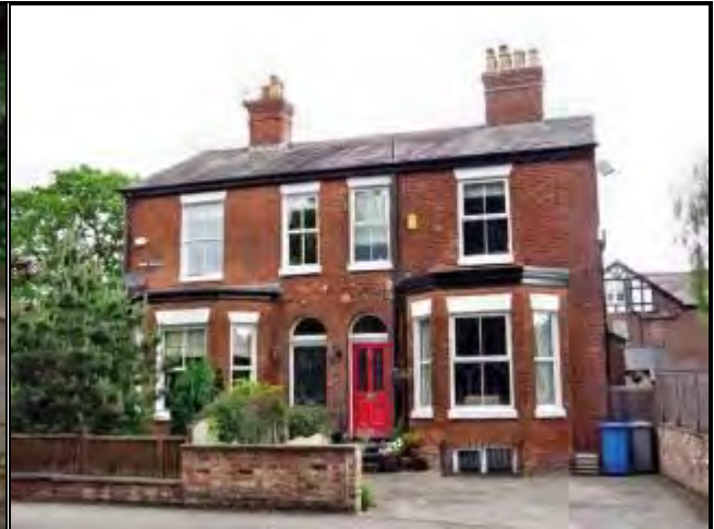
Photograph 114: 3 Park Road, loss of Garden and Gateposts
