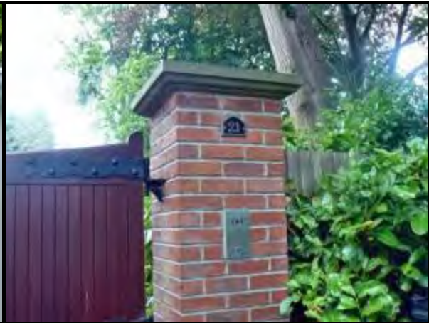
Photograph 106: Modern Brick Pier
