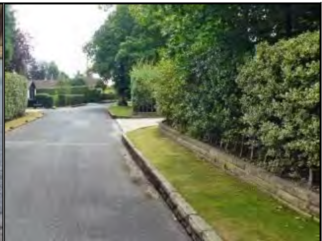
Photograph 128: Patch Repairs along Barrow Lane
