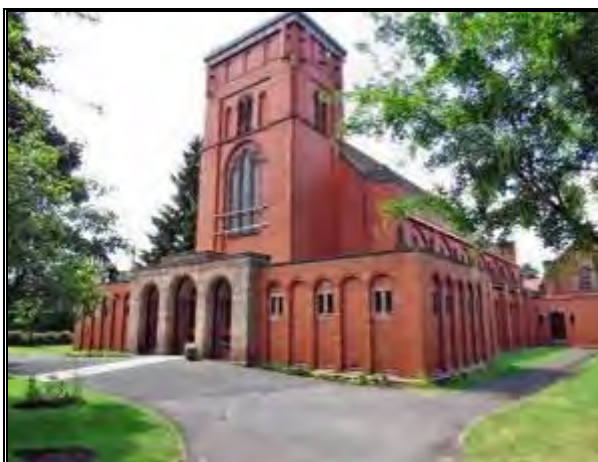
Photograph 38: Open Space around Trinity Hale Church
