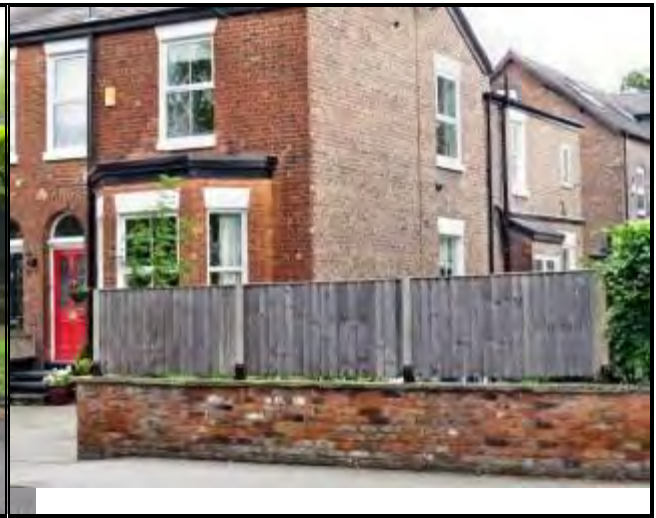
Photograph 120: Brick Wall and Timber Fencing, Ashley Road
