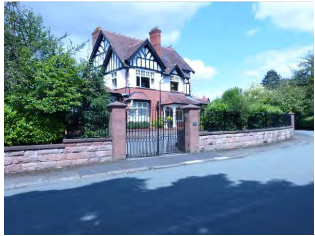
Replacement gate posts on Howard Drive, which are too tall and of an incongruous design. The capping along the original wall is also inappropriate
