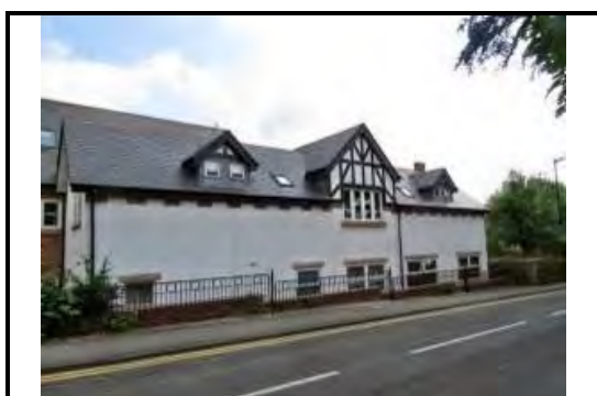
Photograph 35: Former Premises of Hale Motor Company
